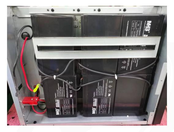
**Step 6:** Use the red and black wires to connect with the red and black terminal (**Be careful! Do not reversely connect the poles)**.
