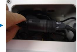
3. Secure the flex conduit fitting onto the junction box hole.
