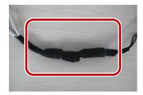
Choose a start point for waterproof tapes and protect the tail cables using waterproof tapes.
