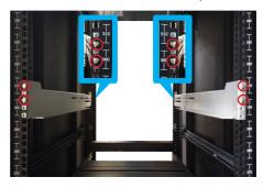
Tighten the screws **>** loosen from **Step 1** on the rails to fix their length.
